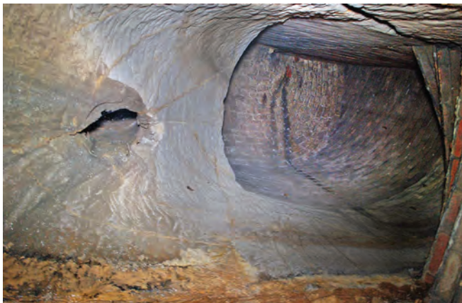
Standing where once there was a wooden staircase, and looking up to a ventilation hole and one-time goods entrance
